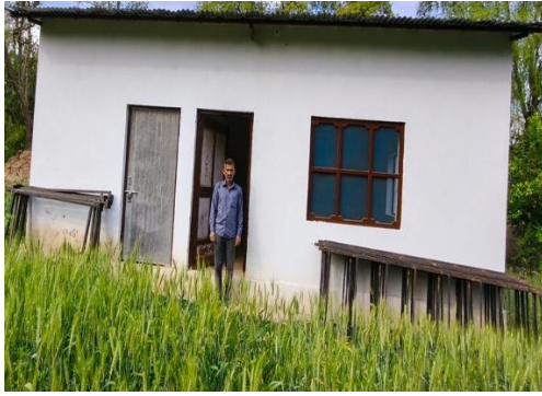
Newly construed rearing house under Silk Samagra-2 & HADP (2024-25).
