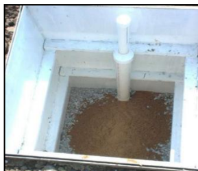
Figure 5: Install the Drain System
