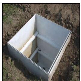
Figure 4: Install the Inner Tank
