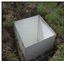
Figure 2: Install the Outer Tank and Backfill Soil
